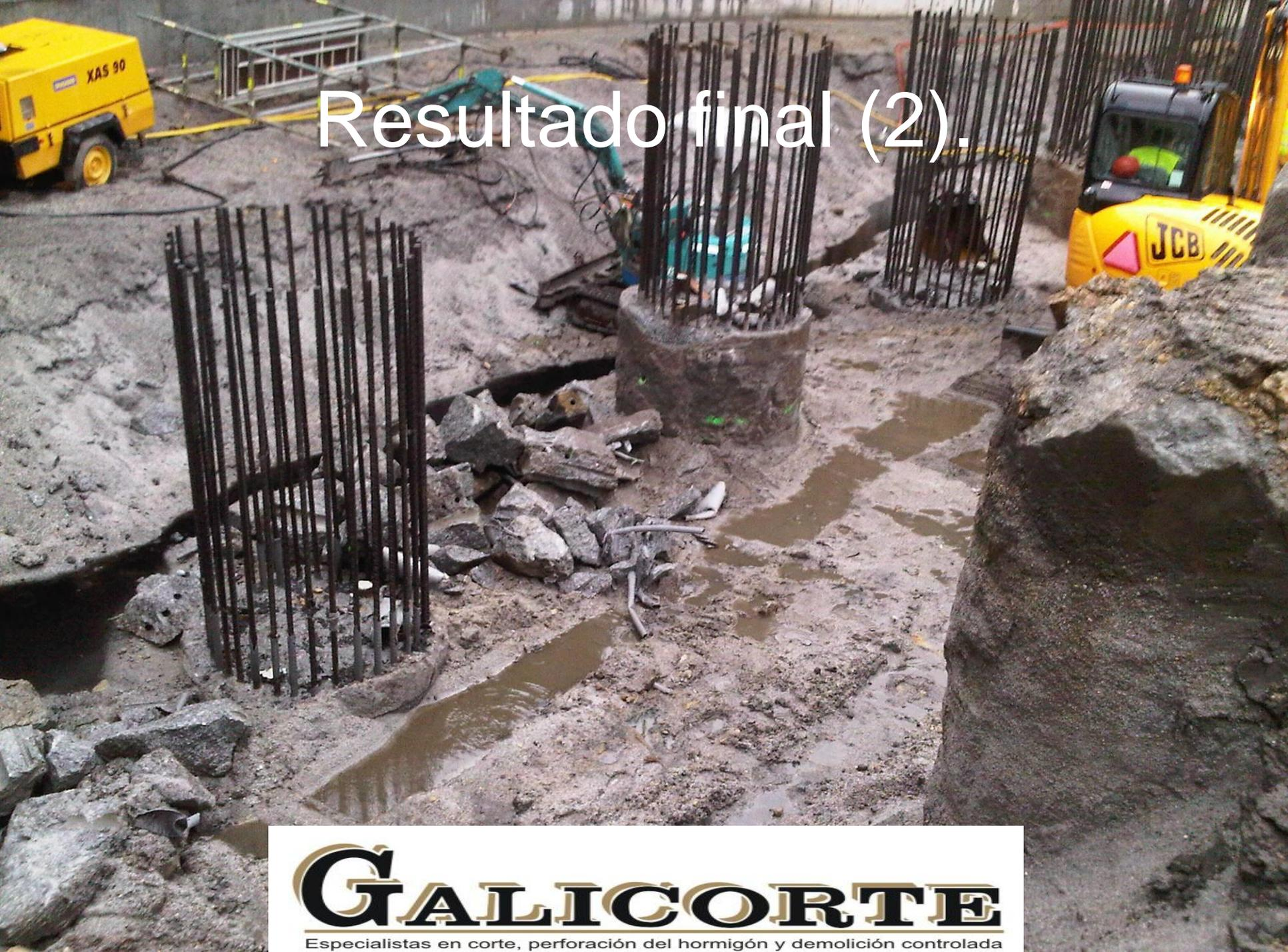
A construction site showing several vertical rebar structures (cylindrical columns) in a muddy, excavated area. A yellow JCB excavator is visible on the right, and a yellow generator or pump unit is on the left. The ground is wet and muddy, with some debris and rocks scattered around. The rebar structures are made of dark metal rods protruding from concrete bases.
