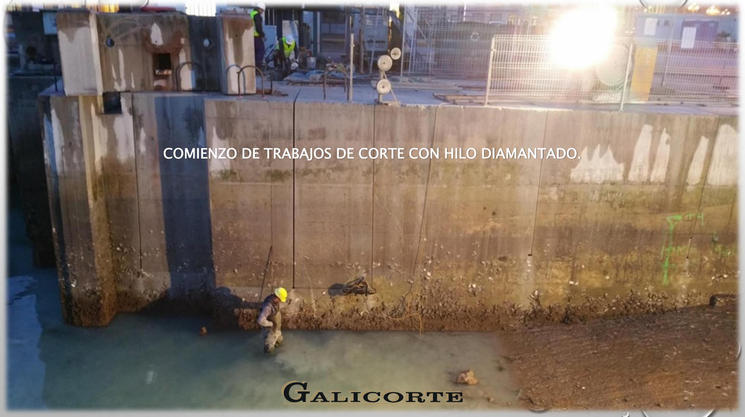
A large-scale construction project at night. A massive concrete wall is being cut with diamond wire. The wall is composed of several vertical panels. A worker in a yellow hard hat and dark clothing is visible at the base of the wall, working with the equipment. The scene is illuminated by bright work lights, creating a high-contrast environment. In the background, there are construction materials, a fence, and some buildings. The overall atmosphere is industrial and focused on the task at hand.
